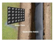
The 7"x1" inner core wrapped with a geotextile fabric and installed in a 3" trench is roughly equal in permeability to a gravel trench 5' wide!
