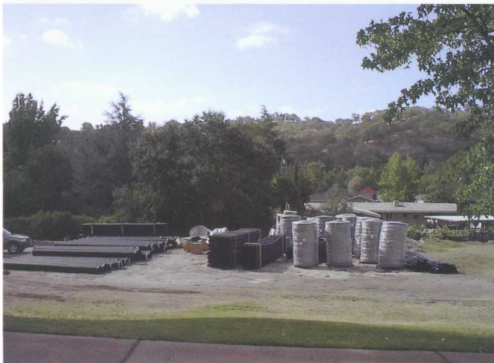
A large staging area allows storage of the new materials for a drainage project.
