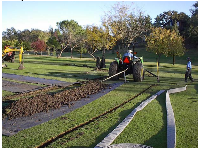
Tarp system for moving spoils
