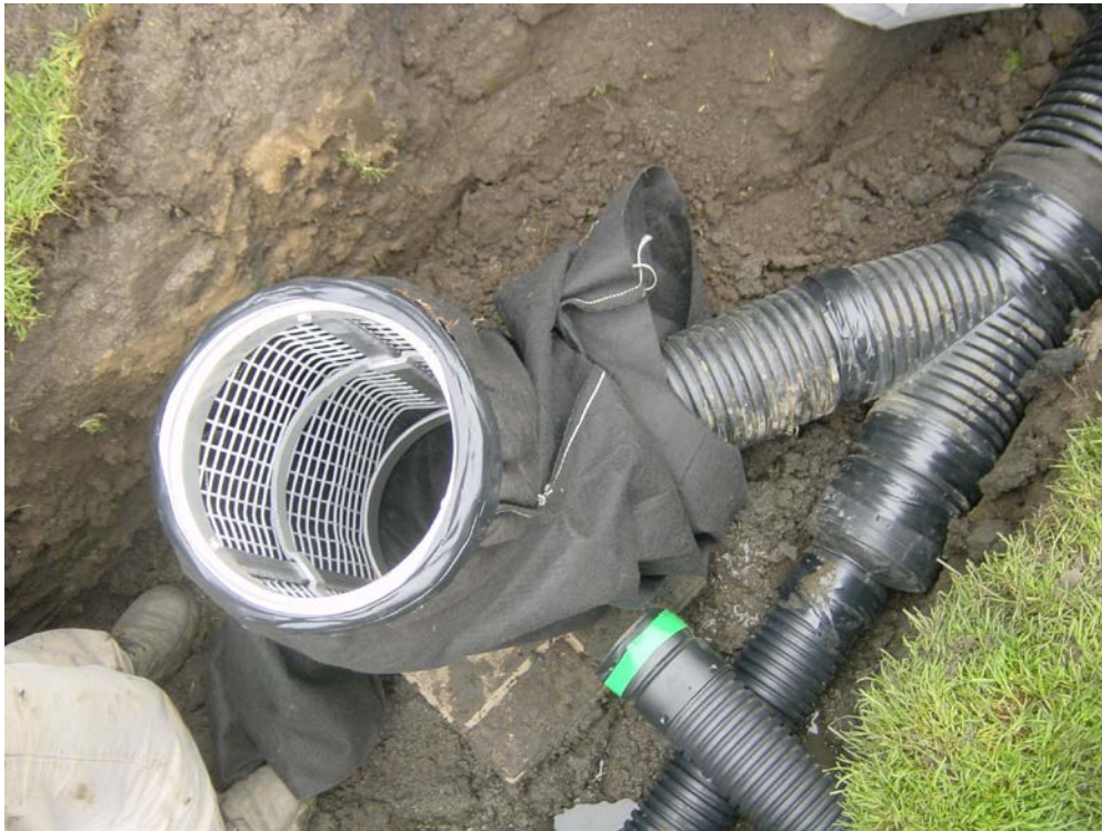
Permeable basin used to collect seepage
