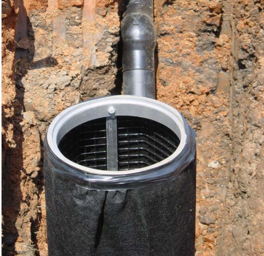
Picture of siphon installation
