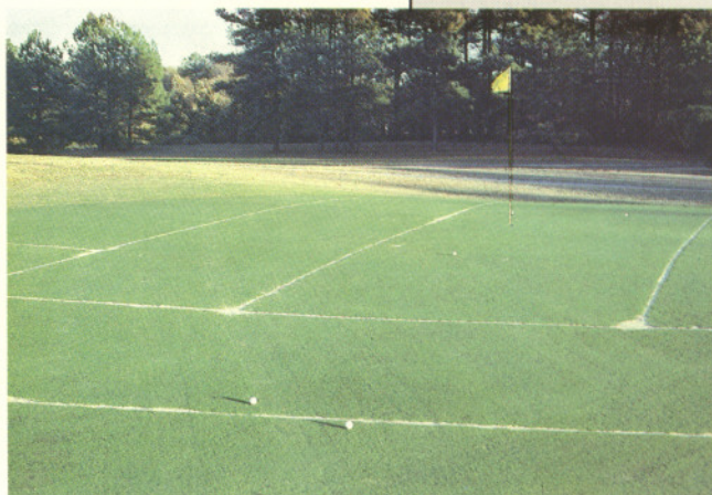
This drain system was installed during a green renovation.
