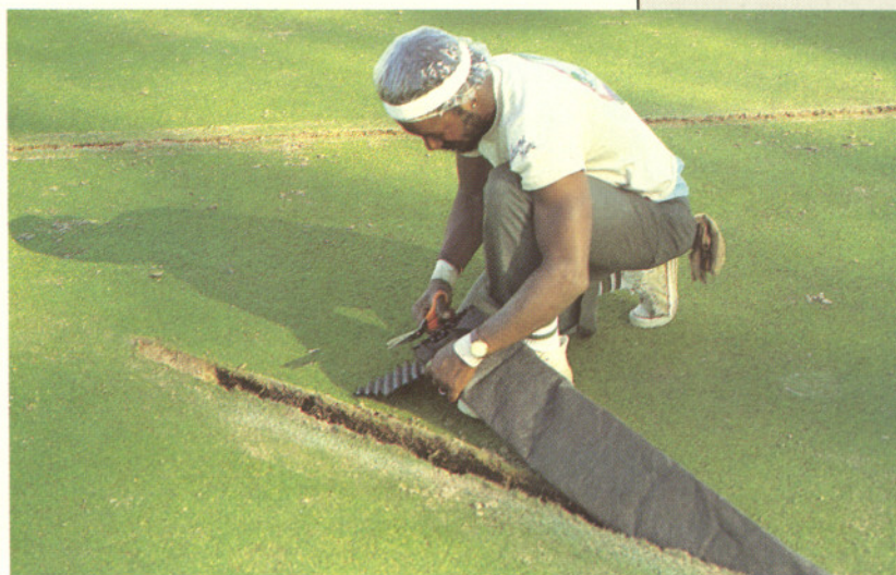
A turf drain was installed prior to backfilling at River Glenn Country Club in Fishers, Ind.
