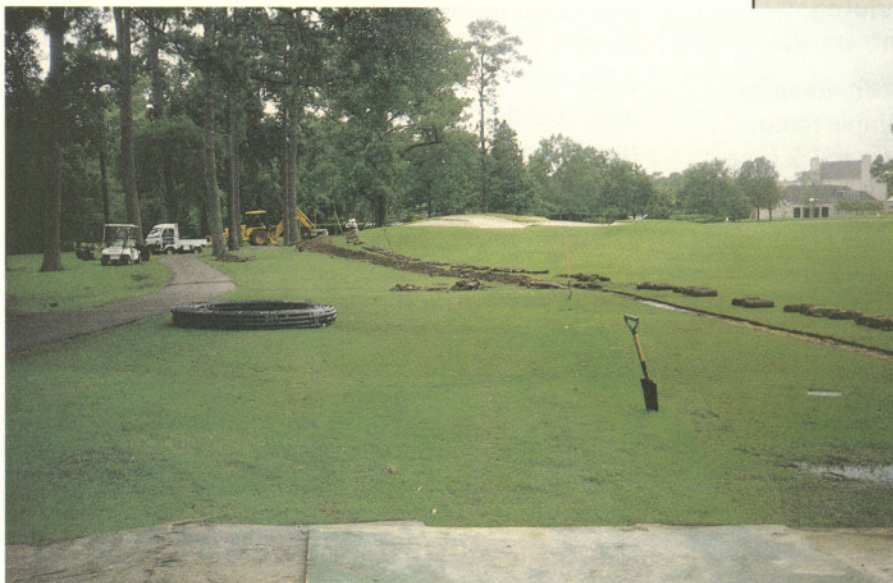
Lines were dug over bunker mounds to a point of relief during siphon drainage installation at River Oaks Country Club in Houston, Texas.
