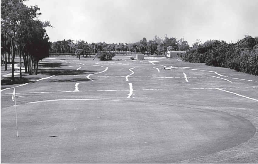
This fairway is divided into several drain fields, with waffle drain lines leading to permeable basins, and then into a siphon system to the relief point.
