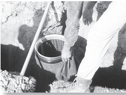
A geotextile-wrapped Perma Basin during installation.
