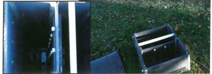
A sliding gate drain (widely used in agricultural fields) regulates the pond depth using a dam principle. (l) View from top (r) gate location relative to pond.
