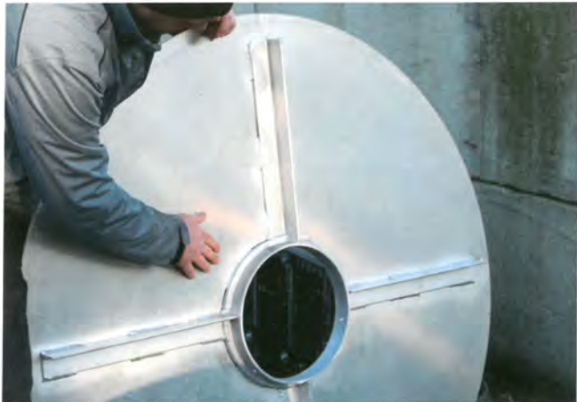
How do you cover a four foot wide sump pit in a playable area? Put a four foot wide lid on it 8" under the soil and grow turf on it. Vent it with a 12" grate.
