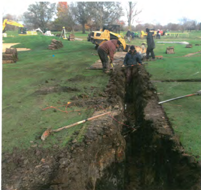
All the soil was removed from each trench cut on the property and backfilled with sand.
